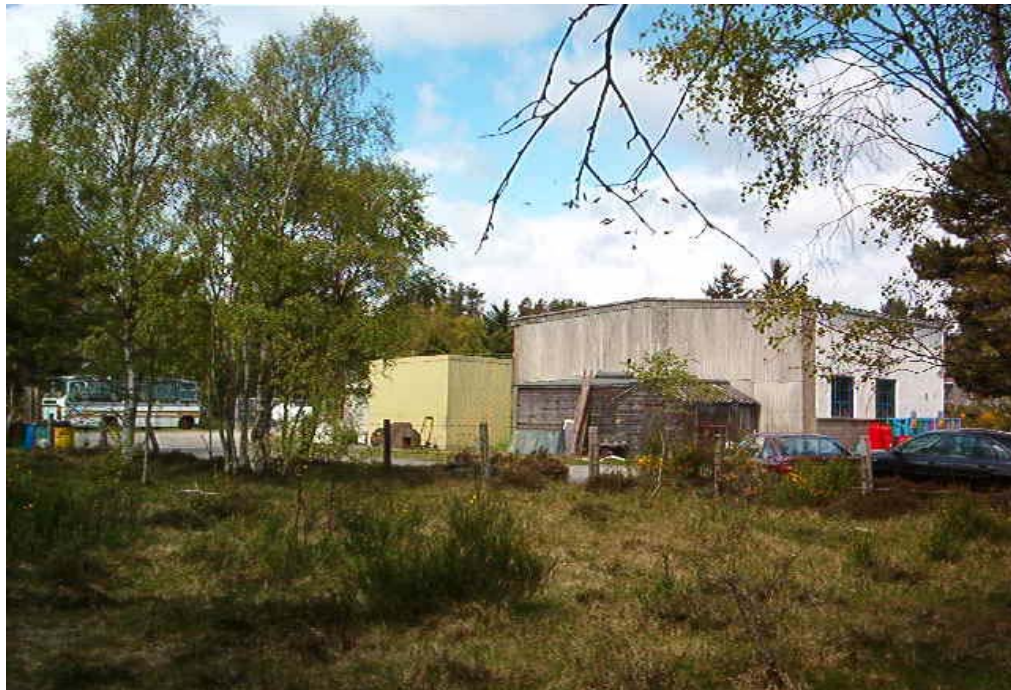
Fig. 3. Rear of site viewed from the woodland to the south
